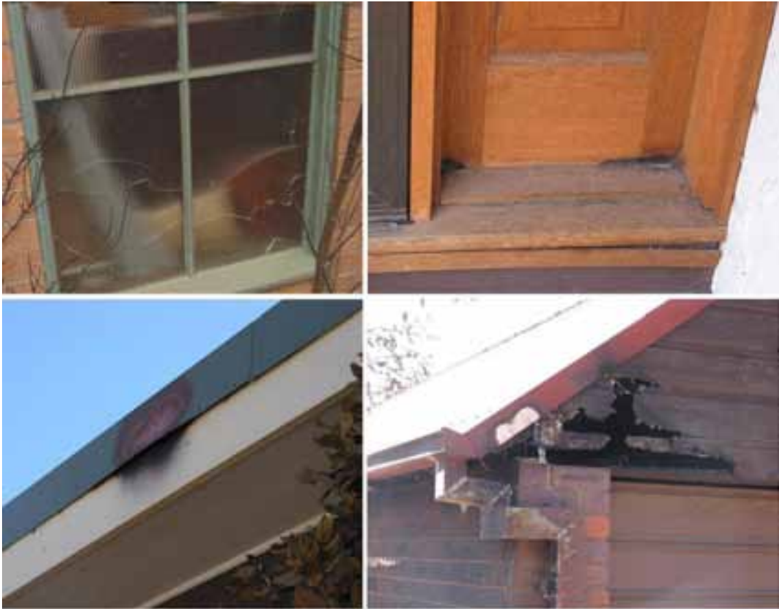
Figure 5. Examples of ember attack on houses in Duffy
